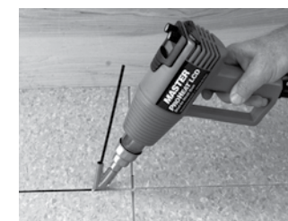
Welding Flooring Material
