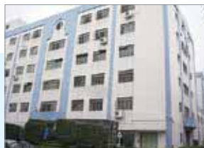
MEAN WELL GUANGZHOU TIANHE R&D CENTER
