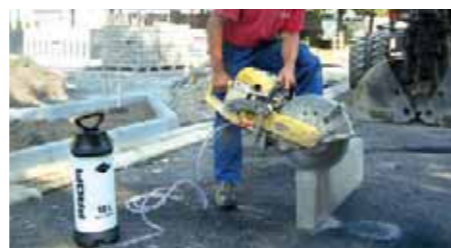
Cut-off grinder in road construction
