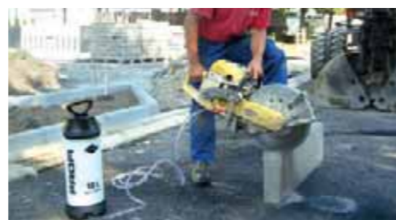
Cut-off grinder in road construction
