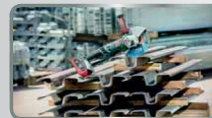
Cutting through 11 crash barriers Material: Sheet steel
