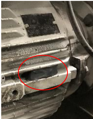
Figure 4: Application of Epoxy
