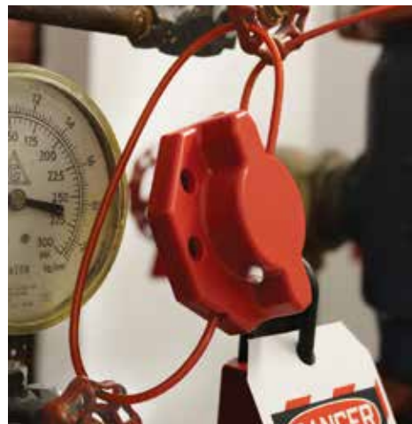
Turn the hasp halves to cinch cable.
