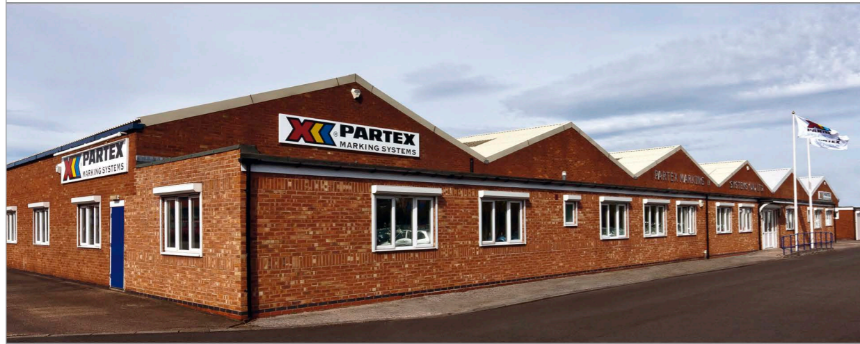
Partex UK headquarters
