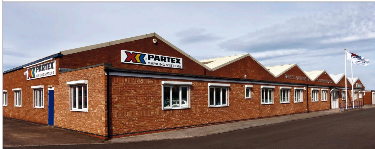
Partex UK headquarters
