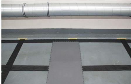
6- First copy the X and Y axis by a line of tiles, this will give you a properly outlined and parallel lay-out:
