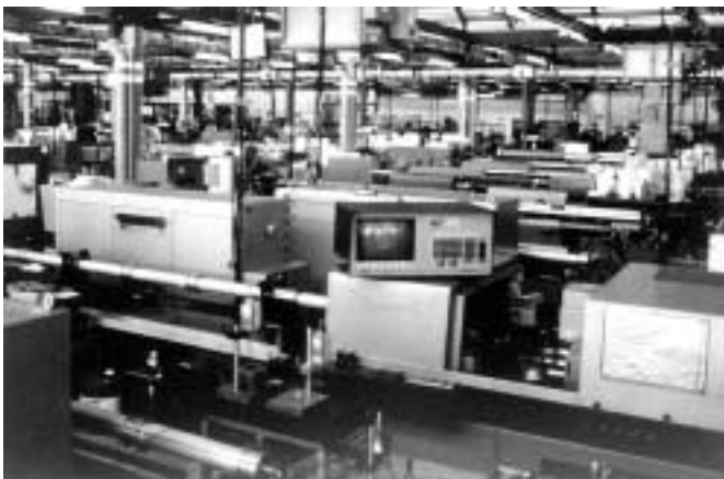
Numerical control lathe
