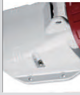
Fastening to exterior wall.
