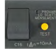
Miniature circuit breakers and residual current (RCBO) 3kA-10mA
