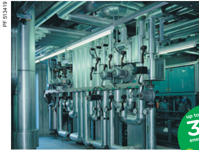
ATV12 controlling a pumping station
