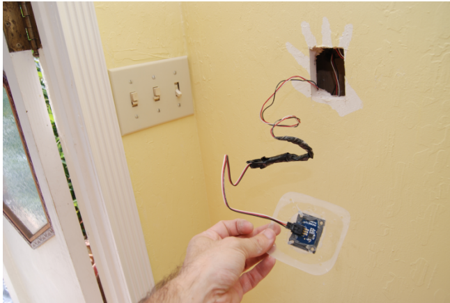
Cut hole in drywall, 1.5 inches x 1.5 inches
