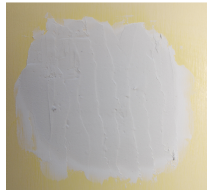
Cover with drywall joint compound
