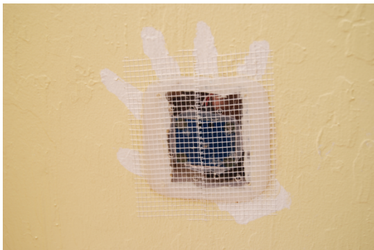
Cover with drywall fiberglass mesh
