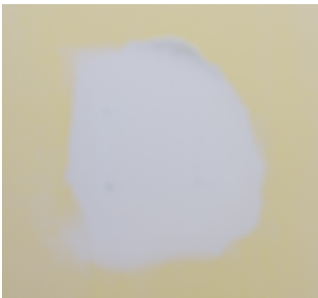
Sand with 150 grit sandpaper. Re-apply joint compound, sand again, and paint.
