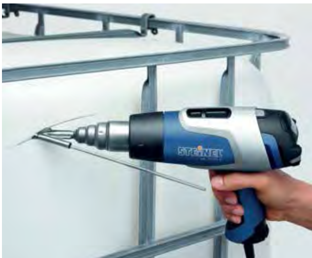
Repairing. Welding PVC water tank.
