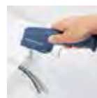
Cutting out small cable channels
