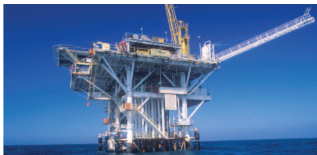
Offshore / Civil Marine
