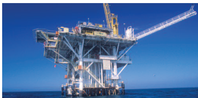
Offshore / Civil Marine
