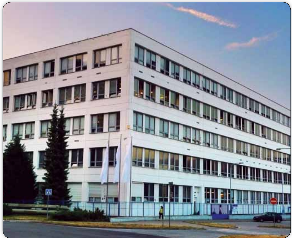
TE Manufacturing Facility in Trutnov, Czech Republic
