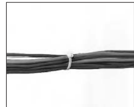
4. Finished tie holds cables firmly.
