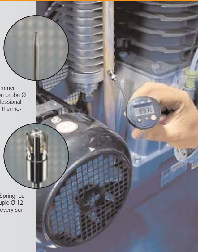
Monitoring the temperature of a refrigeration unit
