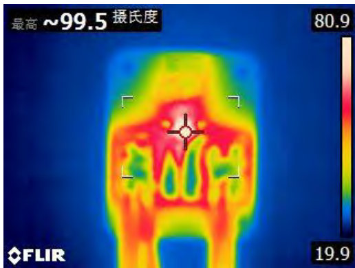
Package Thermography (Input Current 40A)
