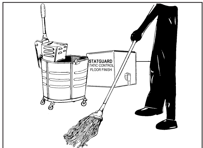
Figure 4. Applying floor finish.
