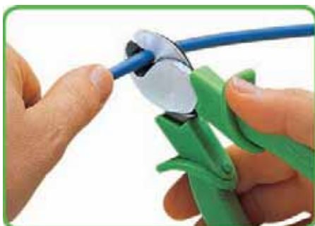
Cutting the cable.
