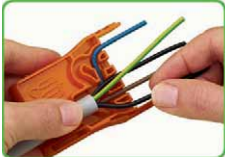
Strip outer insulation, insert cable into the wiring aid and arrange the single wires according to the marking, starting with N.
