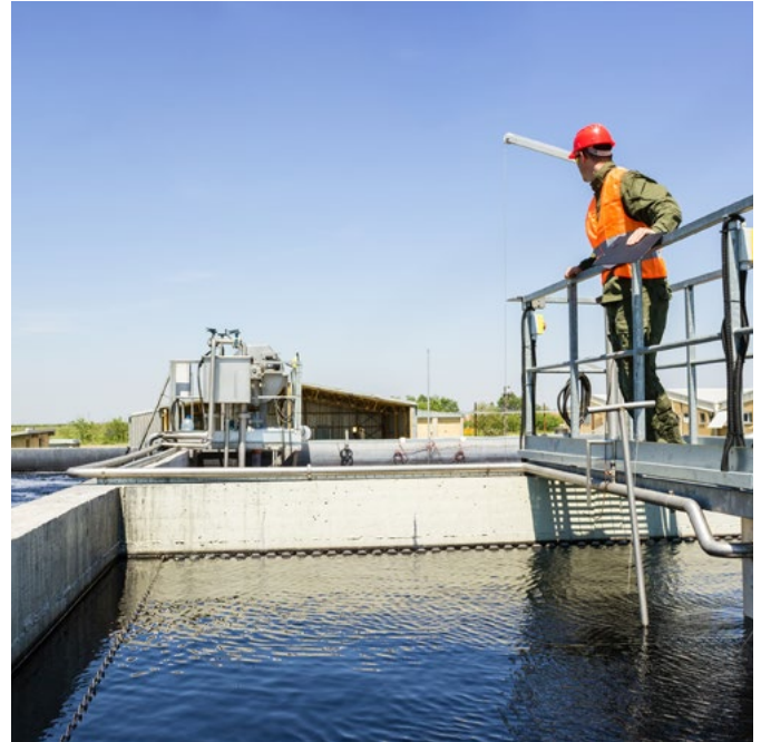
Predestined for emergency shutdown applications: Klippon® Control Stations score when it comes to the safe shutdown of plant sections, such as in the process industry
