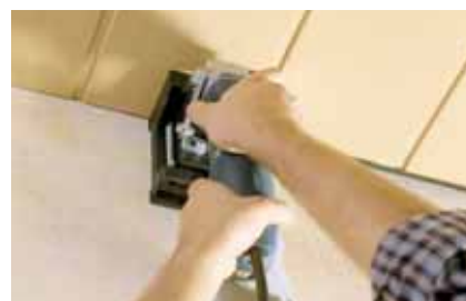
cutting of shadow joints
