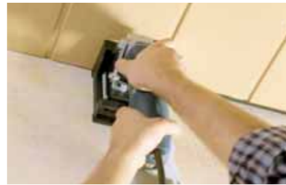
cutting of shadow joints
