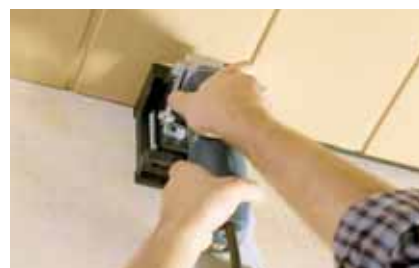
cutting of shadow joints
