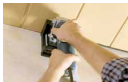
cutting of shadow joints
